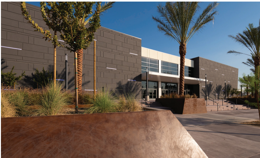
Now located in the Expo at World Market Center
